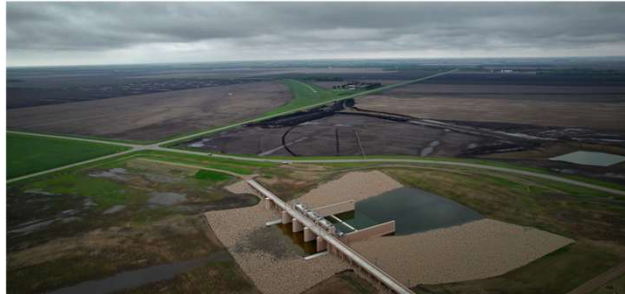
Reach 1B – 29% Completed
