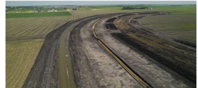
Reach 2A – 76% Completed
