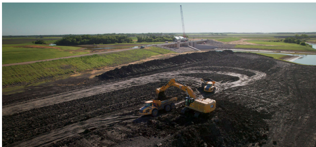
Reach 2B – 37% Completed
