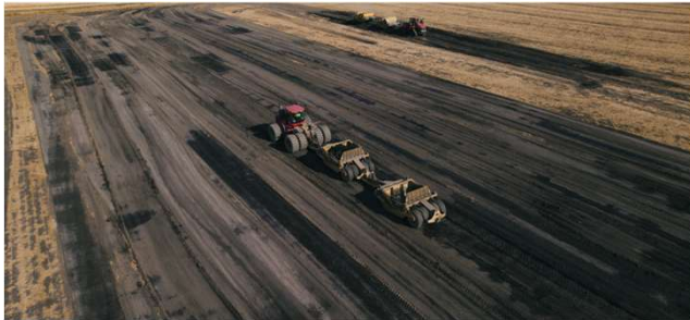
Reach 1A – 100% Completed
