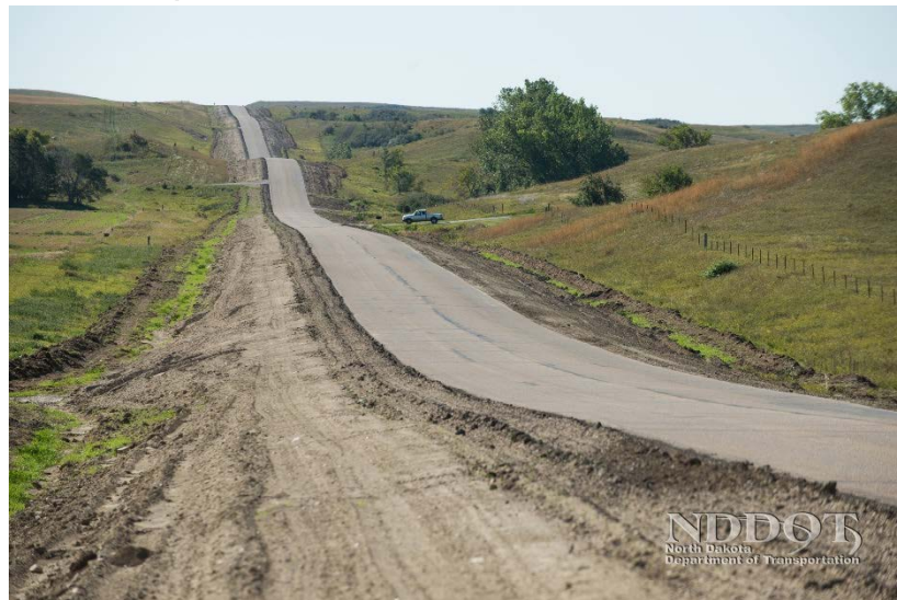
Roadway improvement project in Oliver County.
