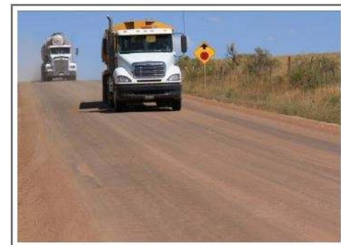
Stable fines preservation on a treated road
